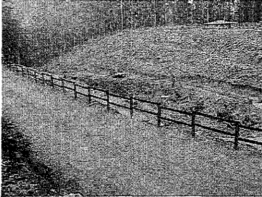
Handrail along the access road
