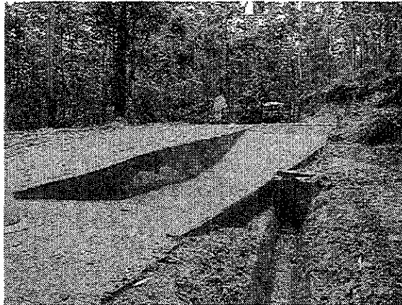
Wheel wash pit
