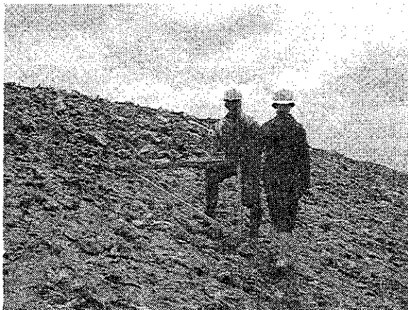
To repair the slope
