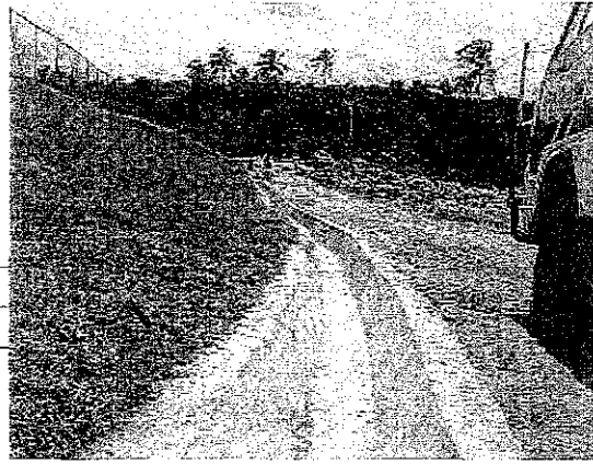
Figure 7-9: Riprap Drain
