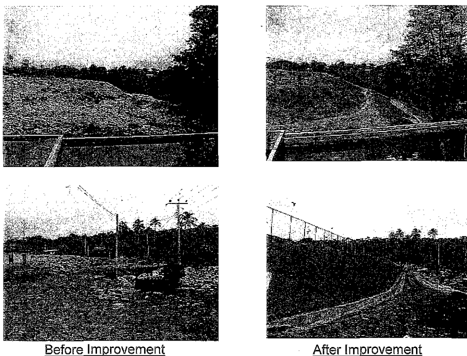
Figure 7-8: Covering Soil and Turfing on the Slope
