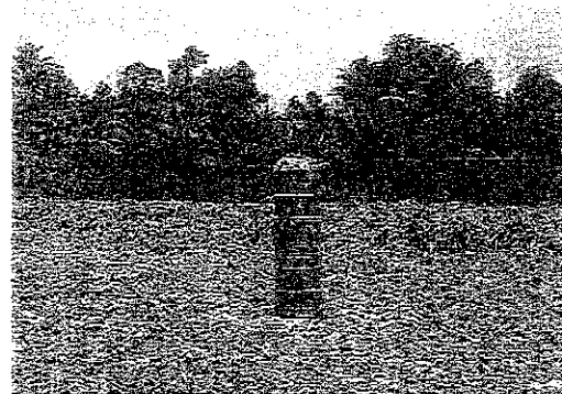
Figure 7-10: Gas Ventilating Facility
