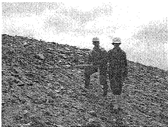
To repair the slope
