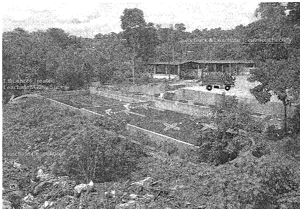
Figure I-4: Image of Leachate Collection Pond and Gully Suck & Leachate Treatment Facility
