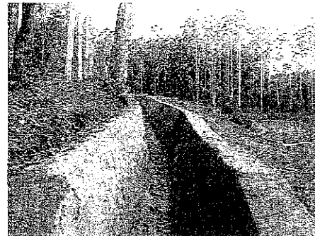
Figure 5-16: Riprap Lined Storm water Drain
