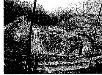
Relocation of existing waste & covering soil
