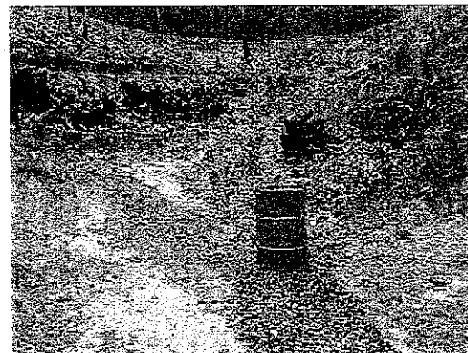
Gas ventilating facility Methane Gas generated by discharged waste is ventilated through a perforated oil barrel which is filled with crushed stone.
