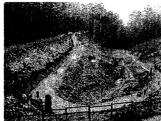
After the improvement The waste dumped was shifted to the lowest area of the landfill site and covered with soil. The leachate collection pipe can be seen along the bottom of the valley.
