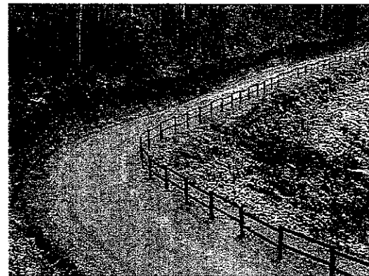
Access road after the improvement The improved access road has ensured that the municipal council can always carry waste to the landfill site even during heavy rains.
