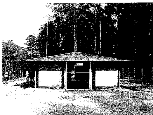
Disposal Pit for Health Care Waste No leachate is generated as all run-off water is intercepted with roofing and drains. The water contained in waste is solidified with cement. The pit is secured by fencing. If the pit gets full, a new pit will be dug and the roof will be shifted there.
