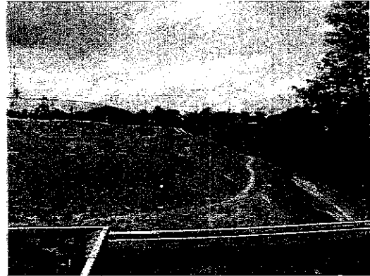
Slope after the improvement The slope was nicely graded, covered with soil and turfed. A fence to prevent waste from scattering was installed along the top of the slope. This mitigated most of the impact and improved view.
