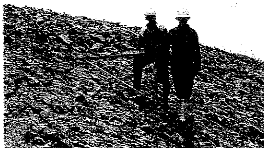
Training of grading slopes The method for grading a slope and turfing was transferred to the counterparts during the improvement because they have to do it by themselves in the future.
