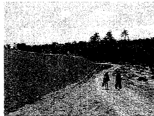
Border after the improvement An embankment was constructed along the edge of the landfill site using waste and it was turfed. People can now walk along the road without noticing the landfill site.
