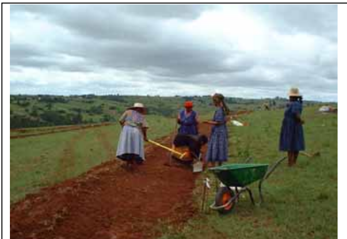
Contour terrace was constructed by community People manually.
