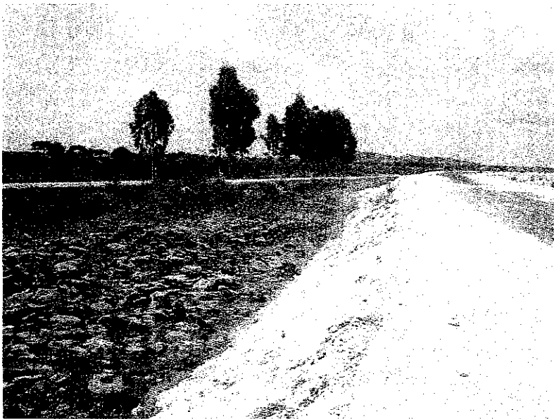
Bypass was constructed to avoid the narrow NR-1.
