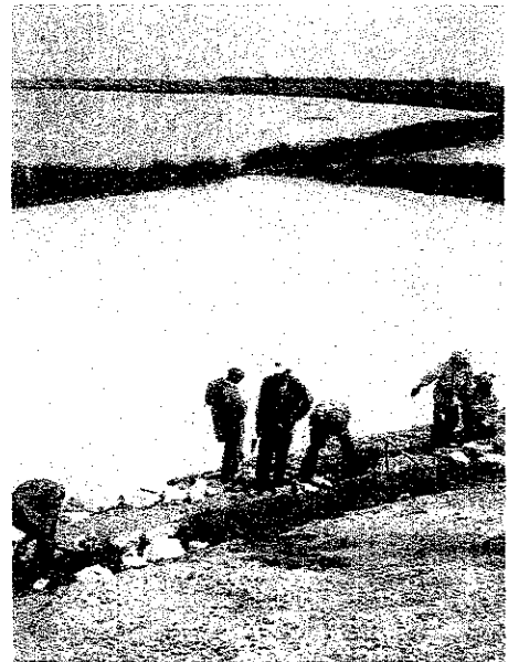
Bypass slope under construction
