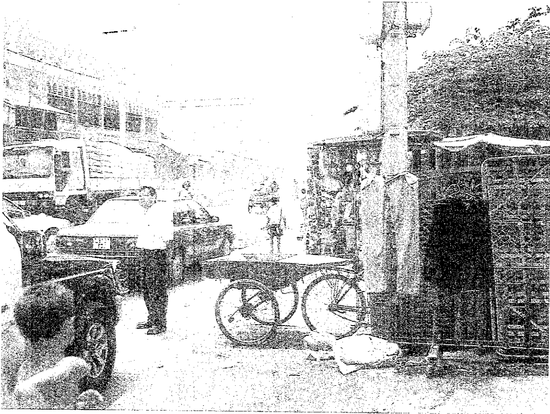
At the most congested portion around Km0+400, many shops and stalls have encroached into roadside, stretching from residential buildings behind. Note that the concrete electric/telegram pole is located only about 7m away from the centerline of the road.
