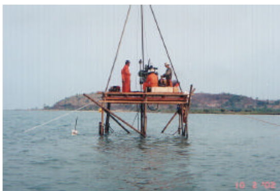
Figure 2-1-29 "Offshore boring, Bojonegara"
