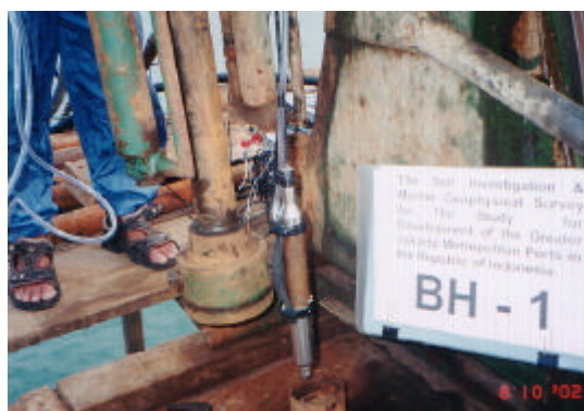
Figure2-1-32 "Geophone to be Lowered into Borehole, Bojonegara"
