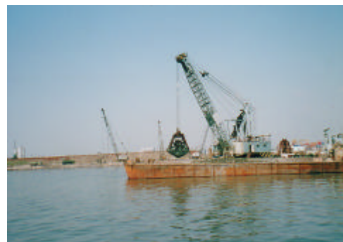
Figure 1-8-3 “Dredging by Grab Dredger, Tanjung Priok Port”
