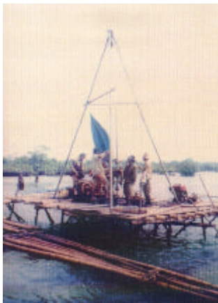
Figure 1-1-14 "Offshore Boring, Tanjung Priok Port"
