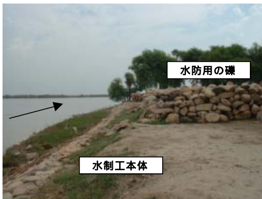
写真-5 堰上流右岸側水制工 (J-Head Spur No.5)
