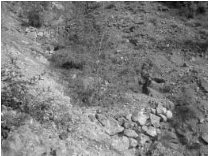
8. Small check dam with Robinia tree planting
