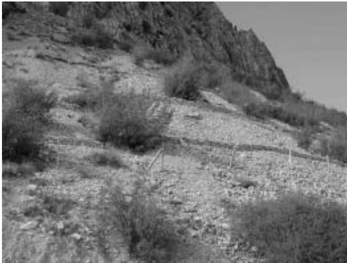
7. Erosion Control: Fencing and terracing by villagers participation
