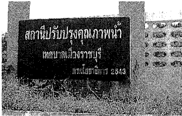
Waste water treatment plant
