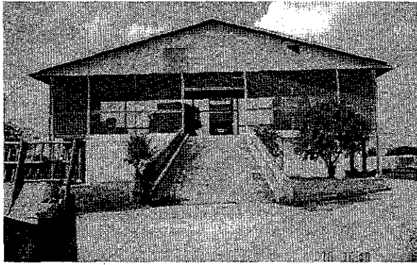
This transfer station has never been operated
