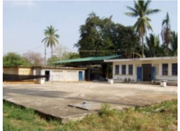
Photo 8 : Clear water reservoir (850m 3 )
