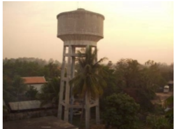
Photo 10 : Elevated tank (500m 3 )
