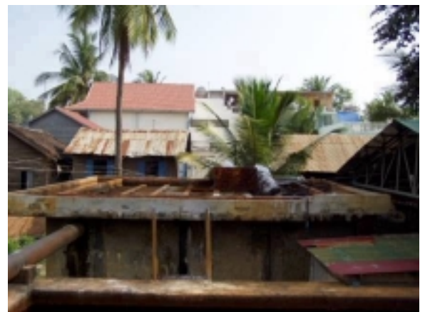
Photo 4 : Aeration tank with pH adjustment by Lime
