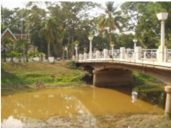
Photo 11 : Distribution pipe on a existing bridge
