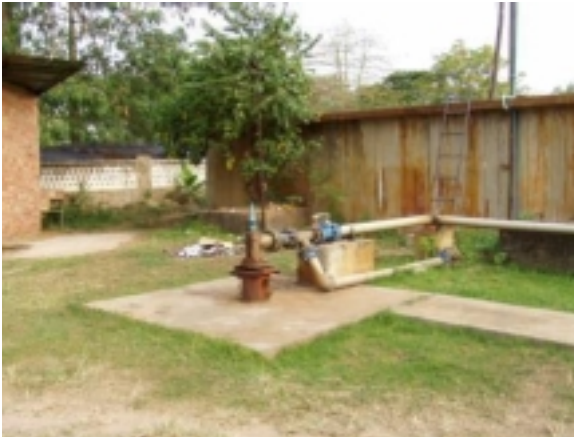
Photo 3 : Raw water Capacity:60 m 3 /hr 18.5 kW
