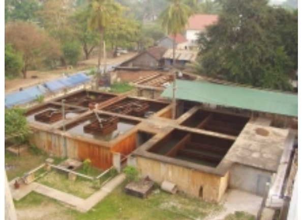
Photo 2 :The existing water treatment plant
