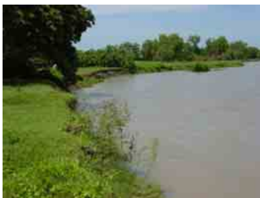
Photo2.3.7-55 Status of the lower reaches
