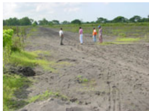
Photo2.3.7-56 Road washed off in the lower reaches
