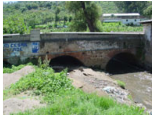
Photo2.3.7.61 Bridge in Postores
