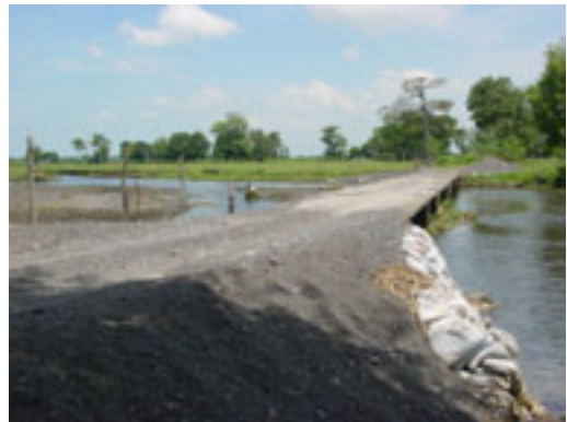
Photo 2.3.4-7 Rivers that diverge from the Achiguate River
