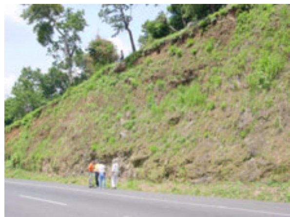
Photo 2.3.7-15 Debris Flow Deposits in Western Part of Escuintla
