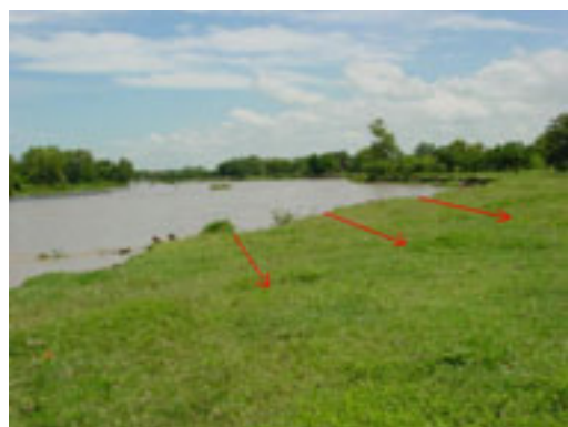
Photo 2.3.4-4 Undercut slope of the Samalá River
