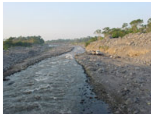
Photo 2.3.5-1 Status of excavation on the riverbed
