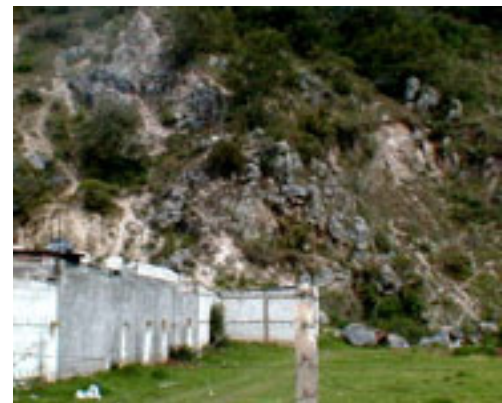
Photo 2.3.7-11 Dangerous cliff at La Pedrera
