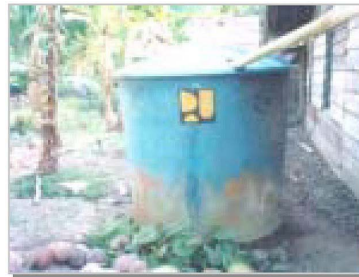
Photo I5.4.1 Domestic Water Tank Provided by SSSIP
