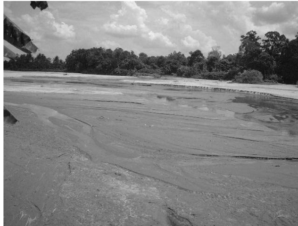
Photo H4.2.1 Sedimentation of the Komerling River
