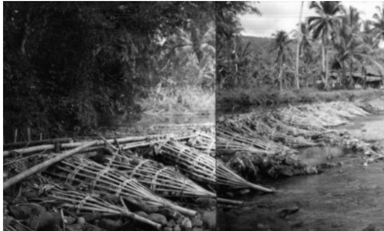
Photo H2.2.2 Bamboo Net Jetty
