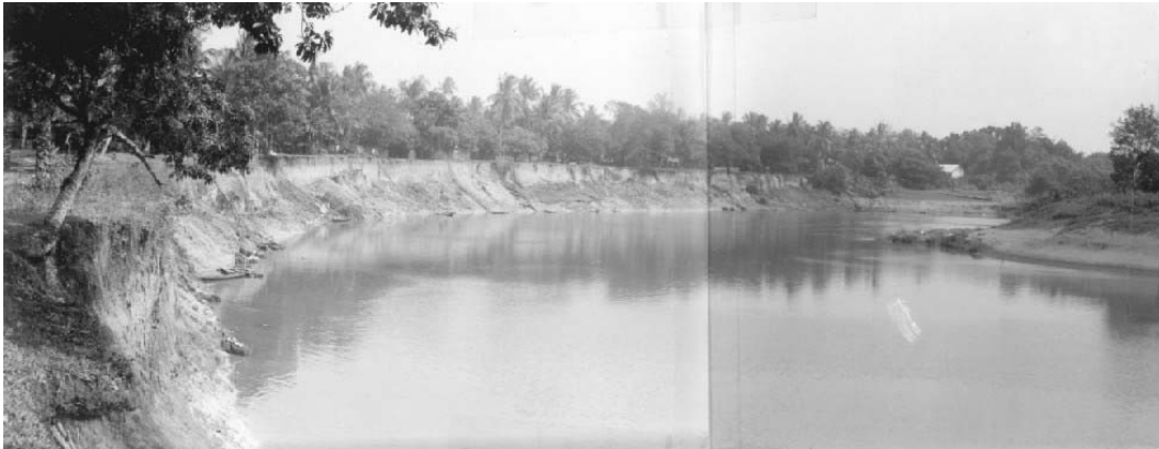
Photo H1.2.1 Bank Erosion at Concave of River
