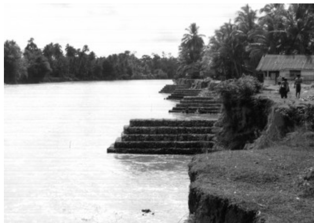
Photo H2.2.1 Typical Gabion Jetty
