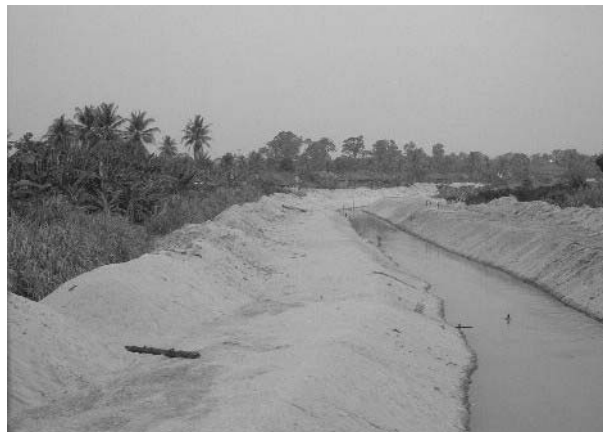
Photo H4.3.1 Dredged Channel
