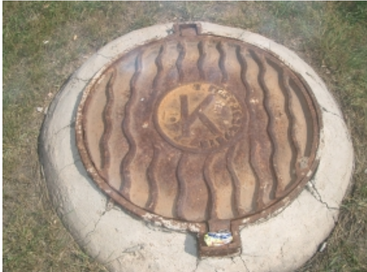
Figure B.15.1 Typical Manhole Cover in " good" condition
