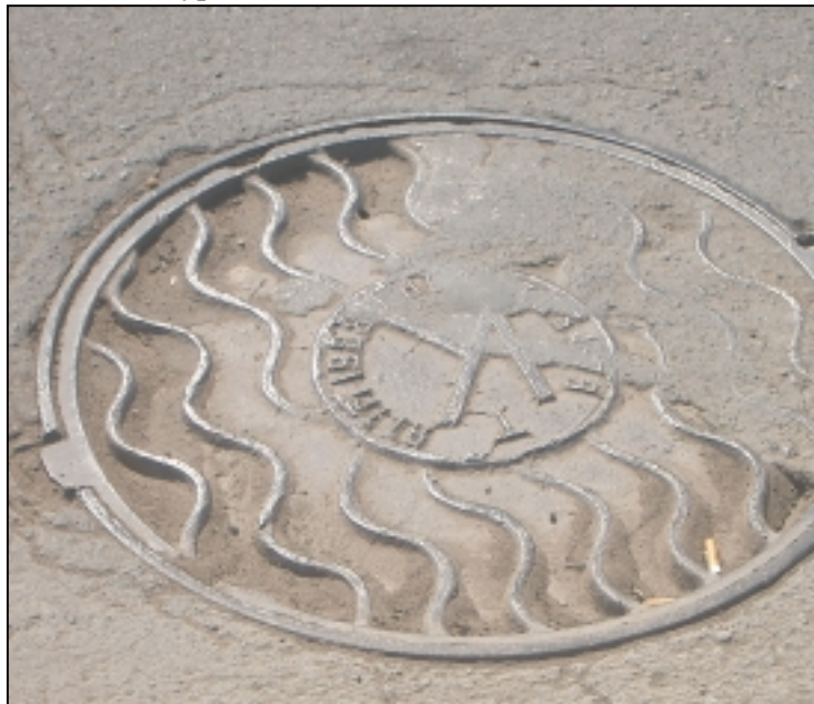
Figure B.15.2 Typical Manhole Cover in " usable" condition on the road
