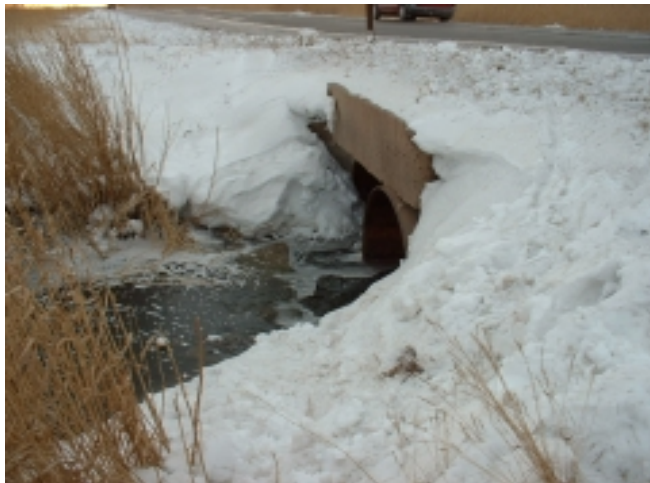
2 culvert under the road
