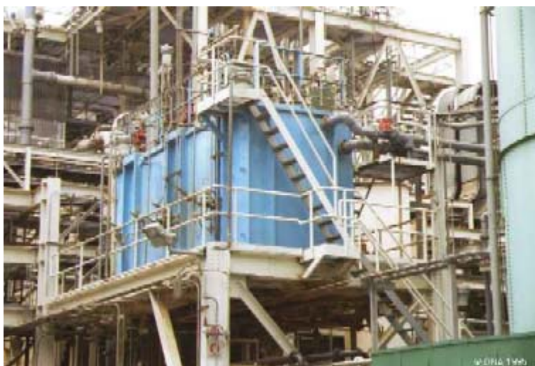
Figure 6.3.15 Example of Continuous Neutralisation / Precipitation Reactor
