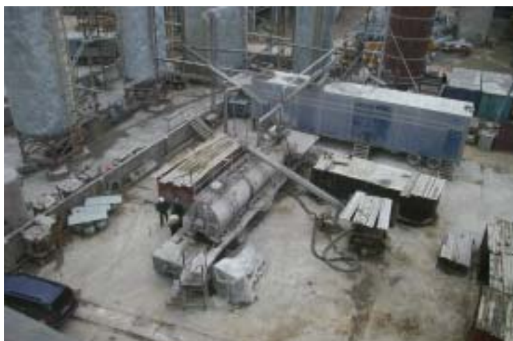
Figure 4.1.1 Sotem Organic Waste Blending Facility
