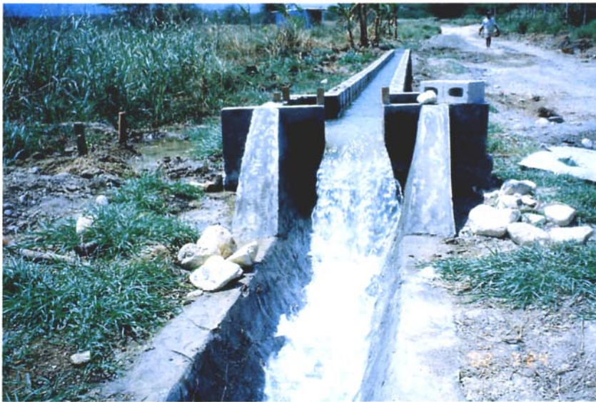
Constructed on-farm irrigation canal in the above project (Expansion of cropping area and improvement of water management were observed)
