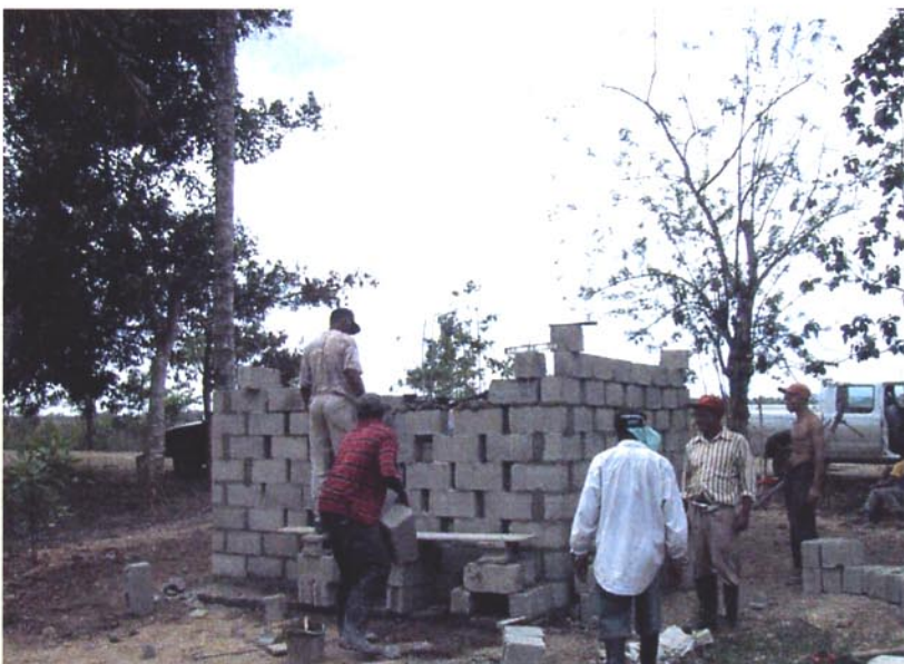
Construction of a pump house by the beneficiary group in the Pilot Project for Domestic Water Supply , La Luisa Model Area
