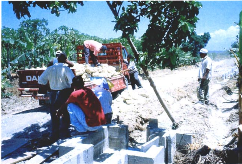
Group D : Tamayo Model Area - On-farm irrigation canal improvement by the Pilot Project for Agricultural Infrastructure Improvement (Labor works and local materials were supplied by the beneficiary group and a truck which is procured by Pilot for Cooperative Reinforcement was used.)
