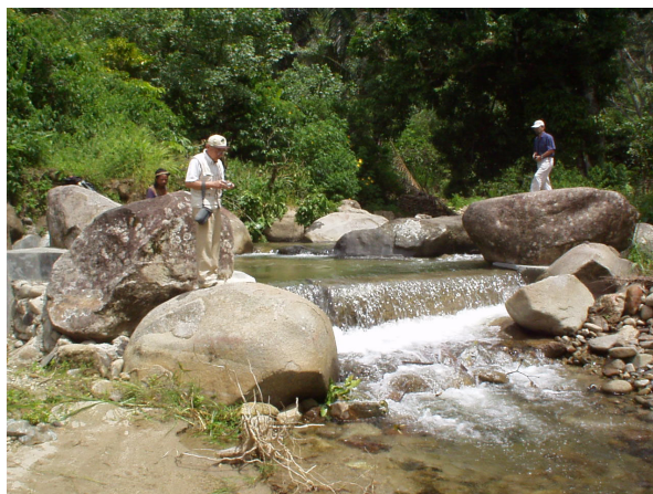
Wet masonry dam
