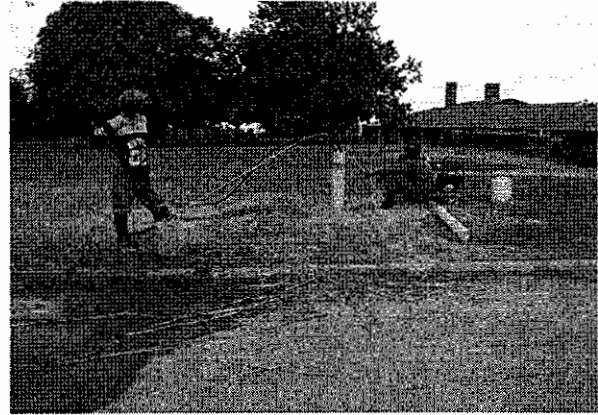
Water Drawing Test from Borehole
