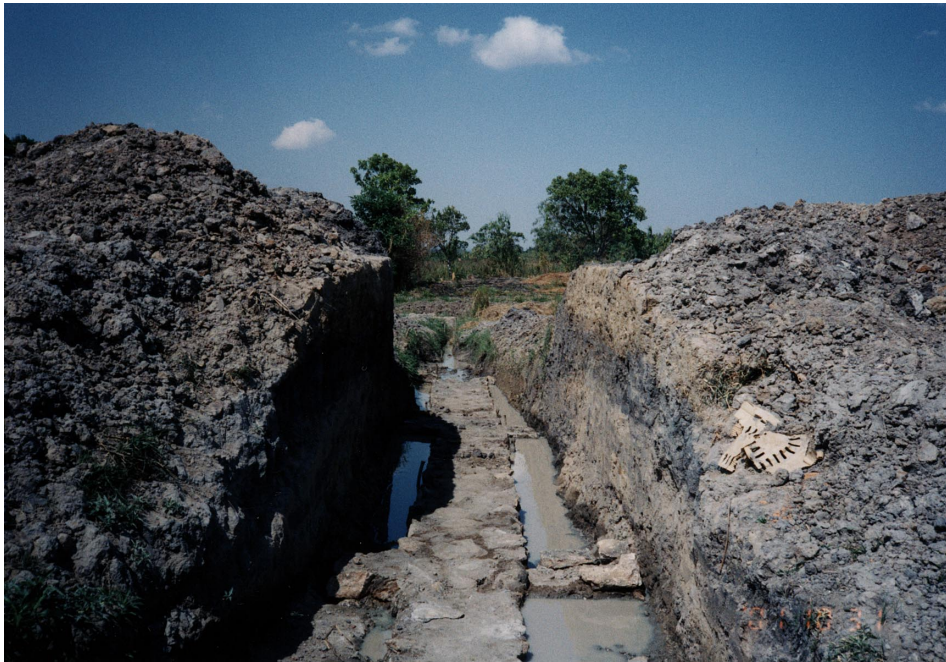
8. KAKHULAJINO DAM DAMBO SELF-HELP PROJECT( DANIDA ) 建設中の取水工
