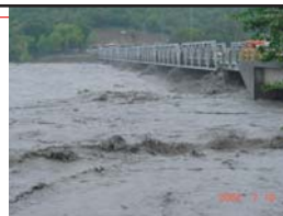
Bucao Bridge (during Flood)
