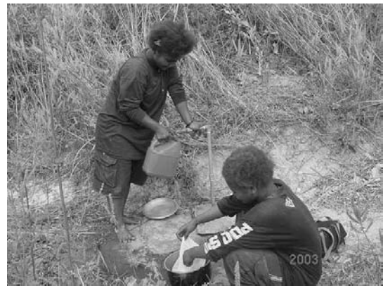
Water supply system for Aeta Community (developed by NGO (ADA) under JICA grass-roots Grant Aide)
