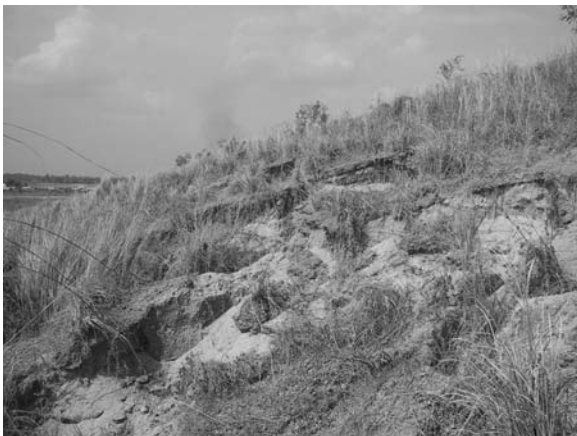
Sta.+17.0 km (January 24, 2003)
