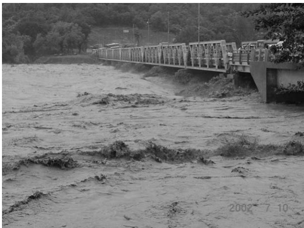
(3) Lahar at the Bucao Bridge (2 Hours after Peak of Lahar Flow)
