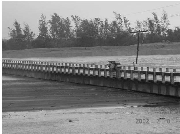
(2) Maculcol Bridge on July 8, 2002
