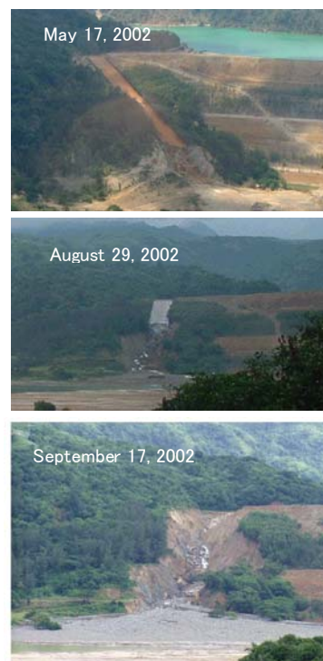
Figure 10.26 Collapse of Spillway of Dizon Dam
