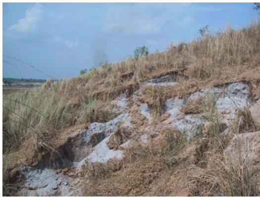
Figure 10.10 Gully Erosion at Sta.17 km
