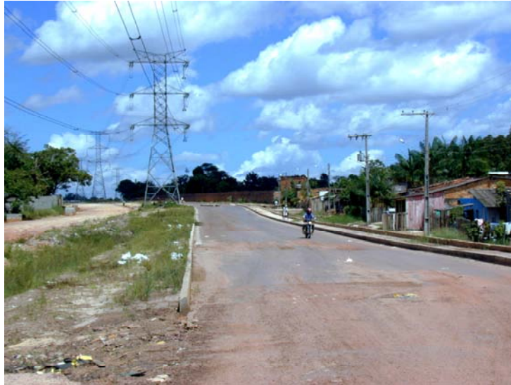
Photo D-5 AVENIDA INDEPENDENCIA Under Construction (Phase II-Section I)
