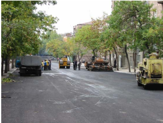
Road Construction in progress
