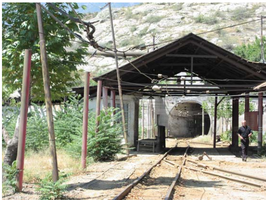
Entrance of Transportation Tunnel
