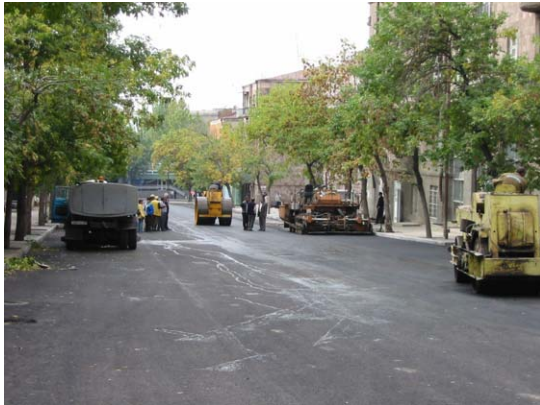
Road Construction in progress
