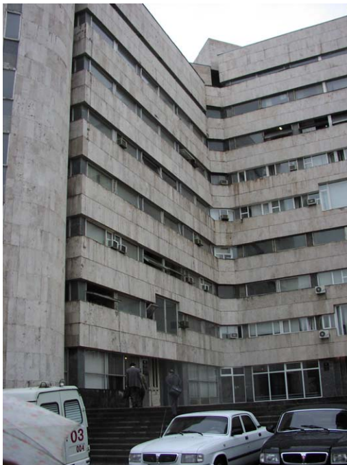
Building of Ministry of Trade and Economic Development
