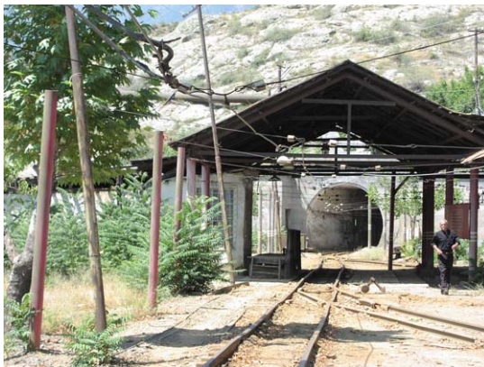
Entrance of Transportation Tunnel
