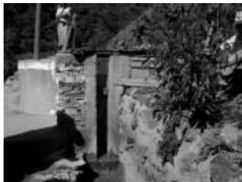
Excess water spillway of Headtank
