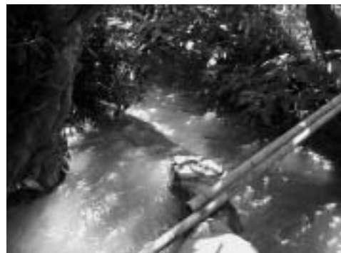
Outfall in operation
