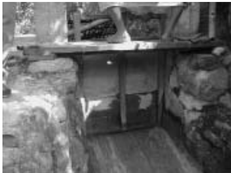
Wooden intake gate
