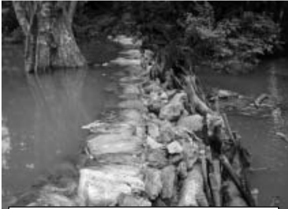
Intake weir with sandbags
