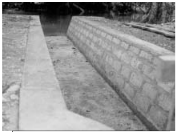
Waterway with side lining with brick
