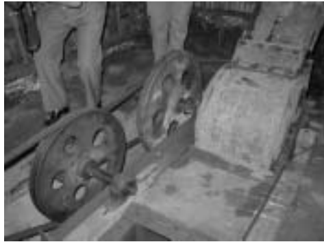
Turbine and belts
