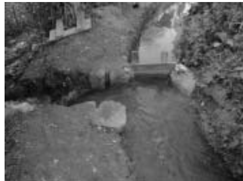
Spillway from Headrace channel
