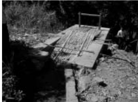
Headtank with bamboo screen
