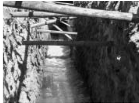
Tailrace channel in operation
