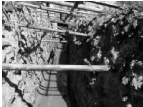
Tailrace channel w/o water
