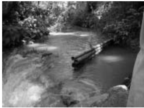
Intake site with debris skimmer-cum-guide wall
