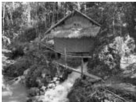
Kyauk Ye Oo Powerhouse
