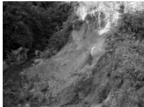
Slope failure below Headrace
