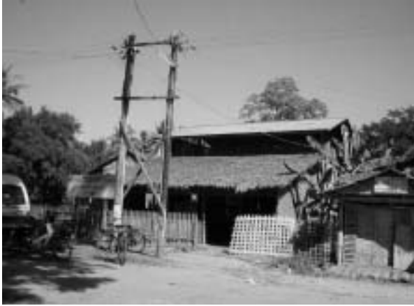
Fig.1 A Building of Rice Husk Gas Engine and Poles for Distribution Lines.
