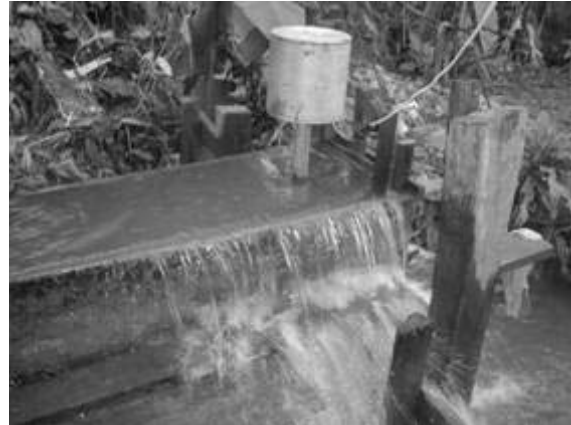
Figure 2 kW Pico Hydro installed behind a tea shop
