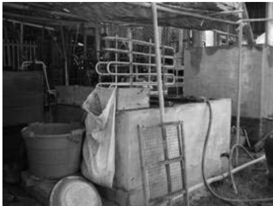
Fig.3 Heat Exchanger of Ice Mill
