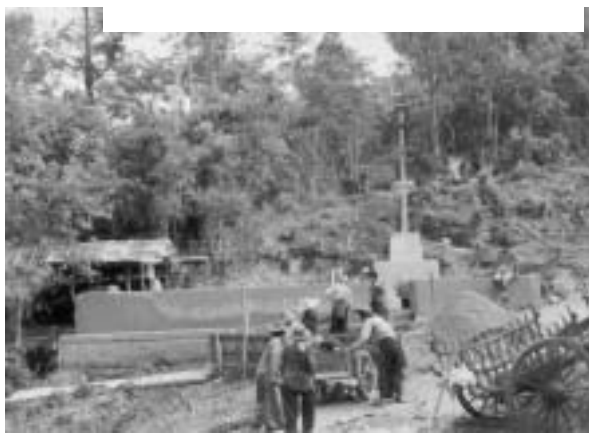
Fig. Installment of Materials by Cow Wheel
