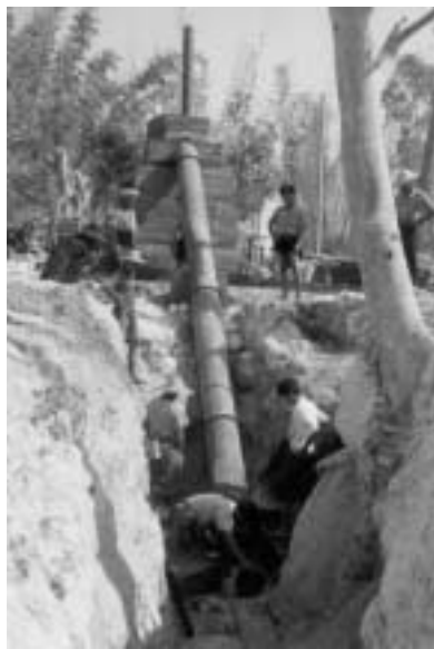
Fig. Excavation and Installment of Penstock Lines
