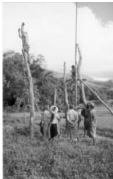
Fig. Wiring the lines of Wooden Poles by Villagers
