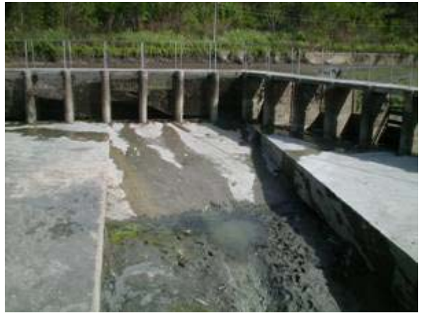
Sloped pond floor towards penstock inlet looking upstream
