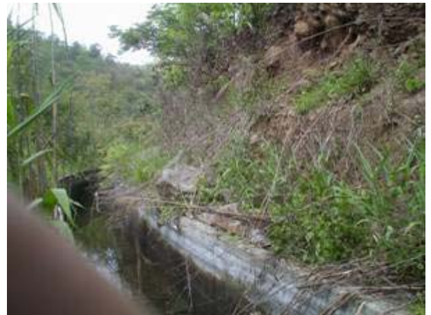
Rock from side slopes
