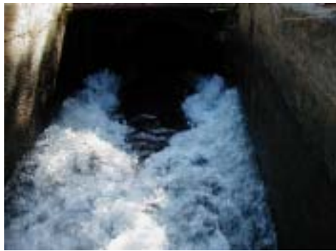
Outlet of Siphon
