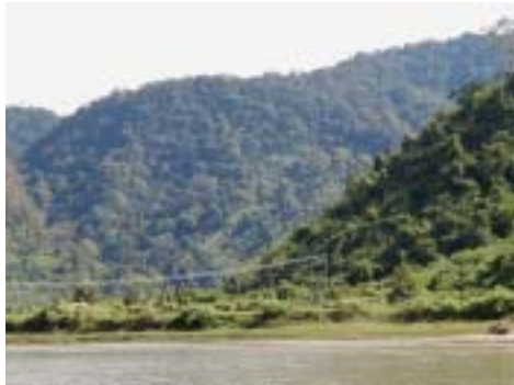
A distant view of penstock
