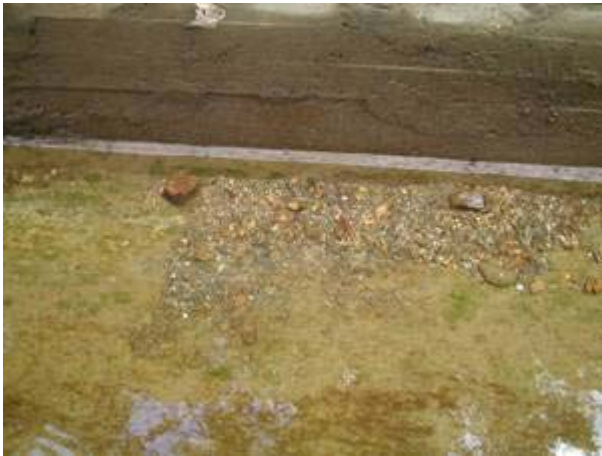
Joint between floor slab and side wall
