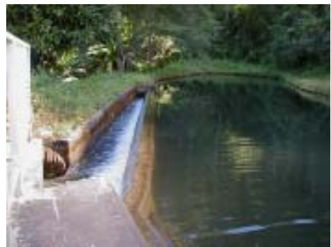
Excess water spillway
