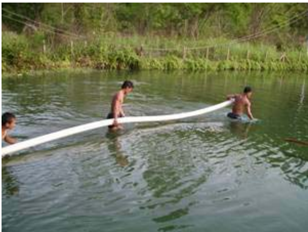
Pipe connection to Flushing head and removing air from pipe
