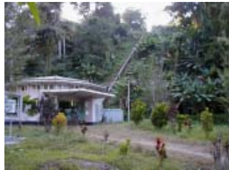
Hopin Power Station & penstock
