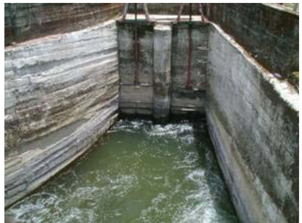
Intake gates looked from upstream
