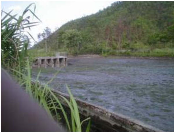
Sediments in the upper part of Regulating Pond, mainly consisting of silt
