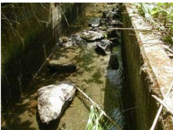
Rock fallen in the channel.
