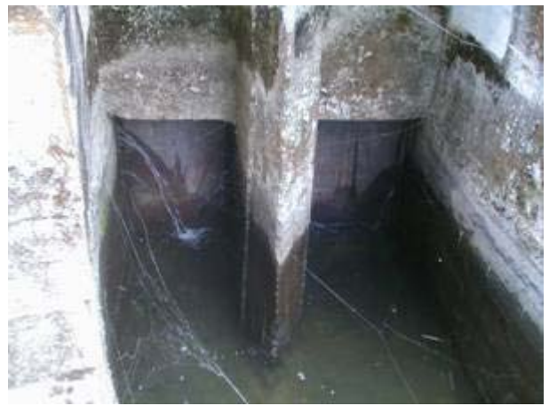
Intake gates fully closed for inspection Water leakage is marginal.
