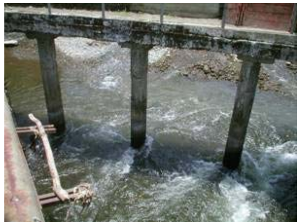
Gravel deposits upstream of the intake
