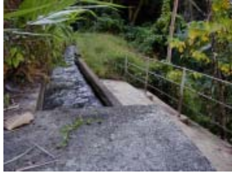
Side-overflow of headrace channel
