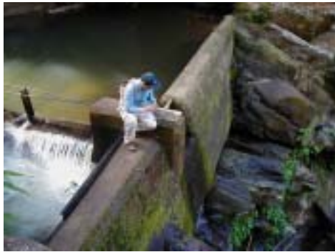
Water flowing into headtank
