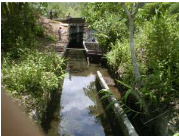
Side spillway section after intake gates fully closed.
