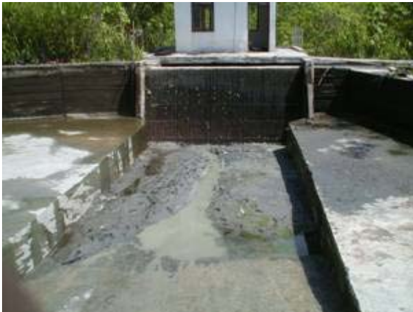
Looking penstock inlet. Sediments were flushed in mid-May 2003
