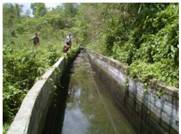
Water pond seen in the curved section is created by dam up effect of the sediments downstream, looking downstream
