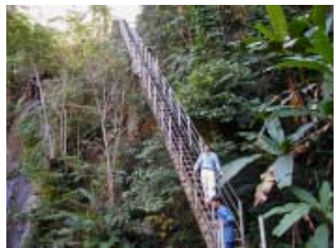
Steps on Siphon Pipes
