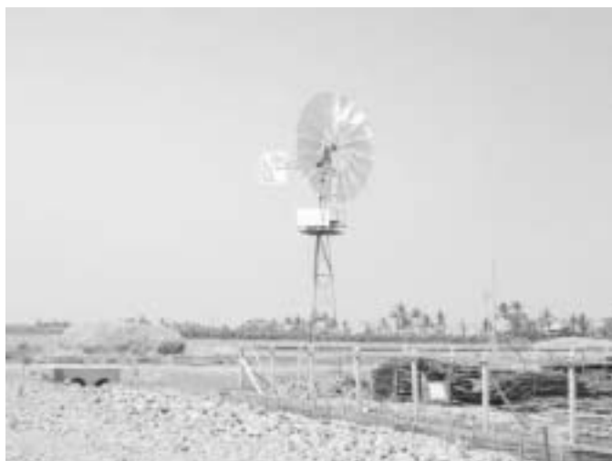
Figure 7 Multi-blade Type Wind Power Generator under Development
