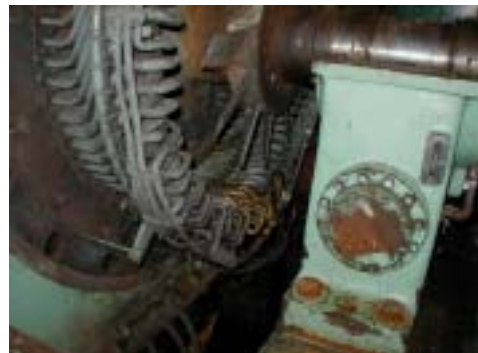
Burnt coils replaced by operators with spare coils
