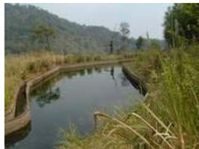
Pondage and approach channel
