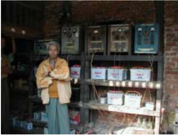
Typical BCS Powered by MEPE Grid in Bago
