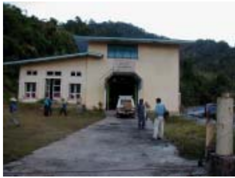
Nam Khan Kha Powerhouse
