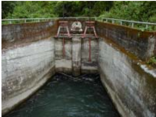
Intake gates viewed from upstream
