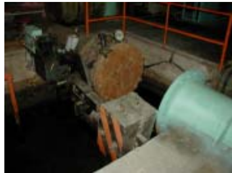
Inlet valve removed for maintenance
