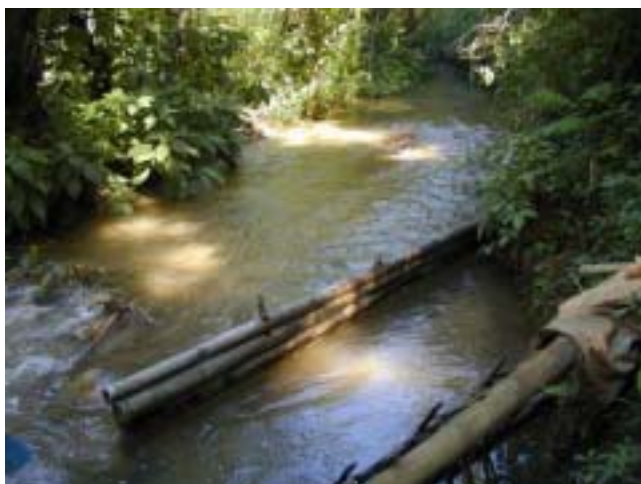
Intake with timber protection
