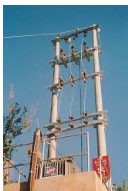
75 kVA Main transformer
