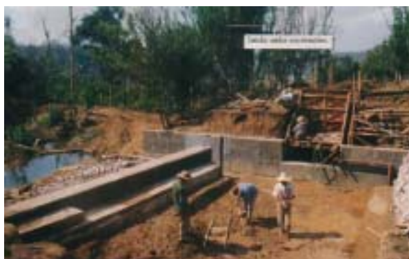
R.C.C weir and intake wingwall work
