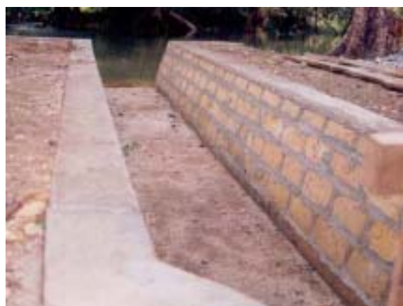
Waterway with side lining with brick
