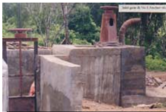
Intake gate and penstock anchor
