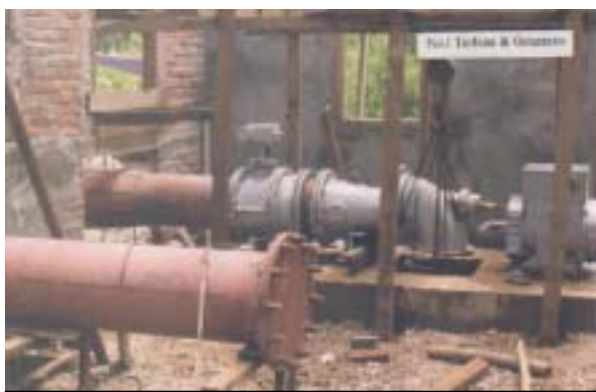
Installation of turbine and generator
