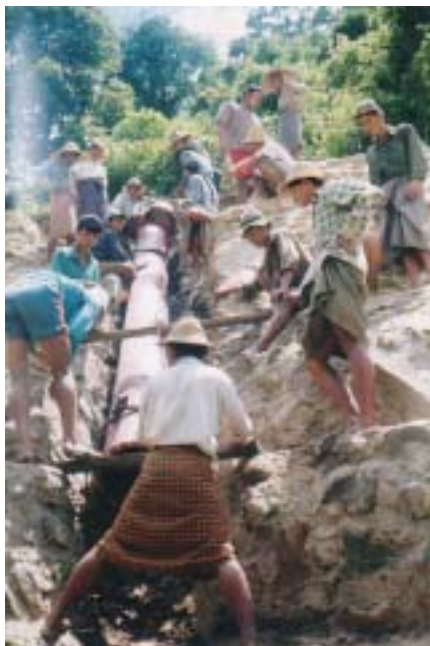
Installation of penstock
