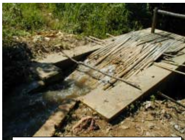
Headtank with bamboo screen
