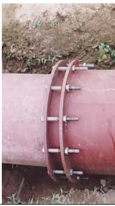
Expansion joint in penstock
