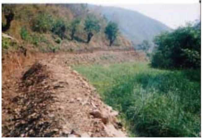
Earth excavation for waterway
