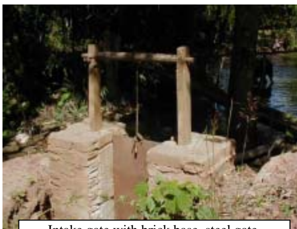
Intake gate with brick base, steel gate, wooden roller and bicycle chain
