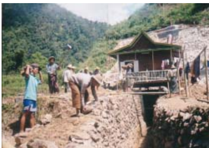
Tailrace excavation and lining
