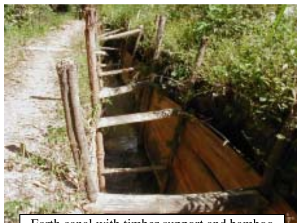
Earth canal with timber support and bamboo side wall protection
