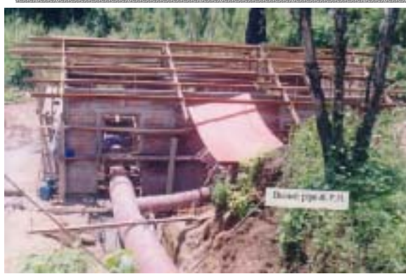
Powerhouse and penstock branch
