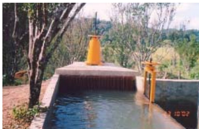
Concrete-lined headtank and waterway
