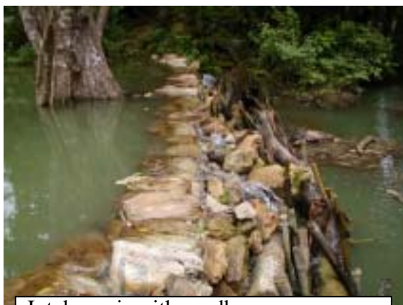
Intake weir with sandbags
