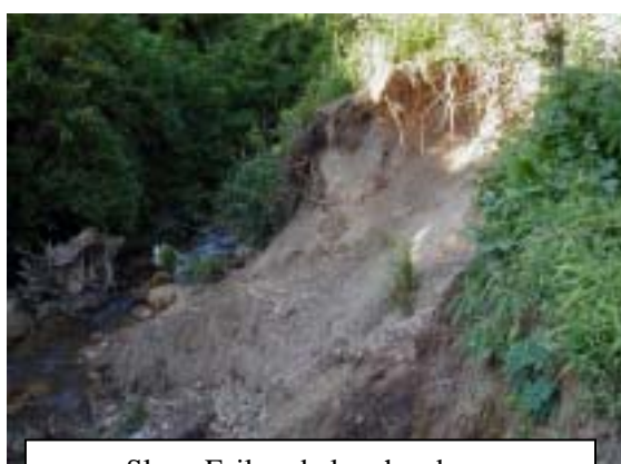
Slope Failure below headrace
