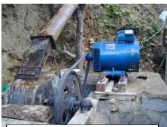
Penstock end with reducer, turbine, and generator
