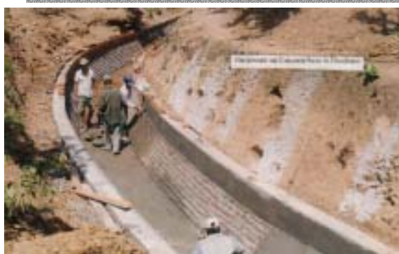
Brickwork for the base of headrace
