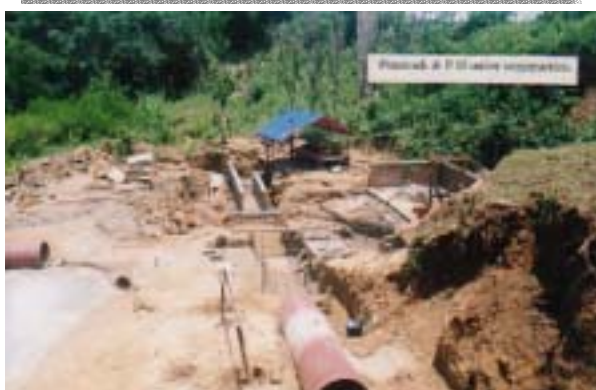
Penstock and powerhouse construction
