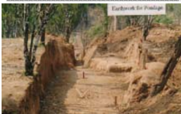
Earthwork of headtank and canal
