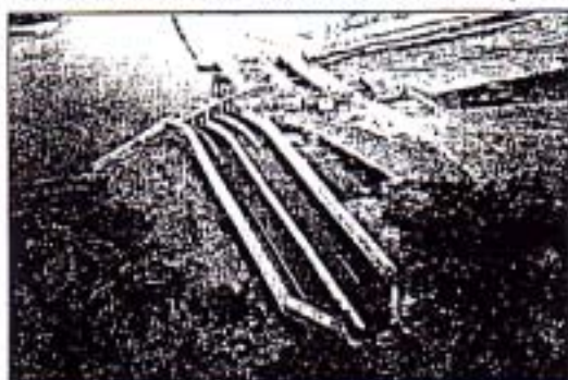
A Serpent Sediment Sluicing System at the 12 MW Jhimruk hydropower project in Nepal.
