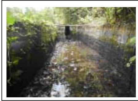
Figure 4.3.2 Sediment in Headrace Canal
