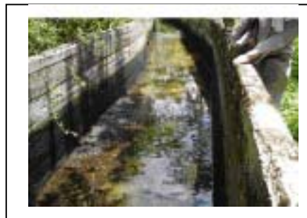
Figure 4.3.4 Floor Slab at the Leakage Section
