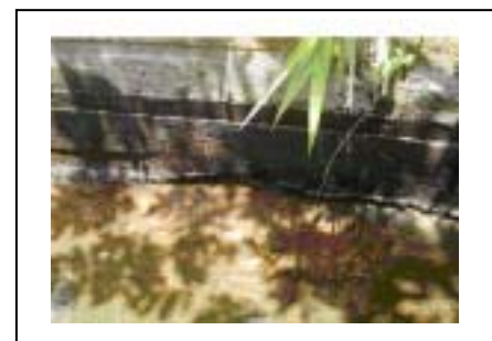
Figure 4.3.7 Erosion of Foot of Wall
