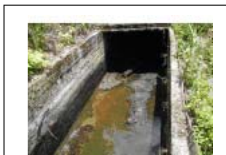
Figure 4.3.6 Erosion of Floor Slab
