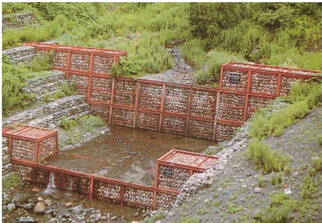
Figure 4.3.21 Steel Frame Gabion
