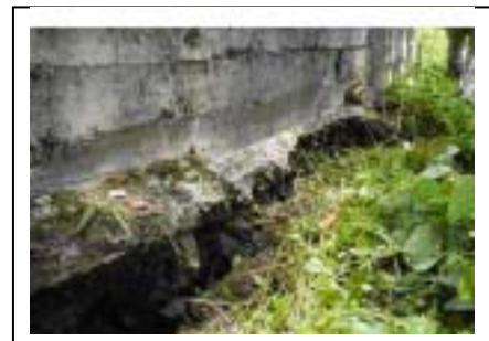
Figure 4.3.5 Outside Conditions of Foundation at the Leakage Section
