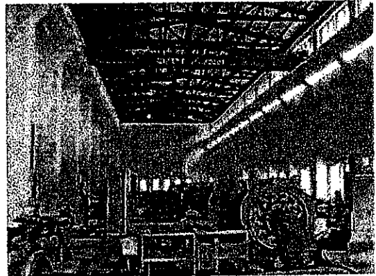
Turbine &amp; Generator
