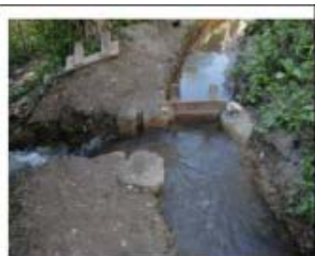
Earth Canal with Bypass
