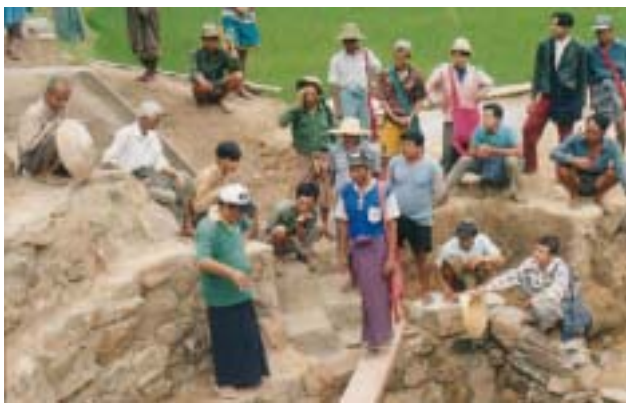
Construction on Self-Help: Waterways - Power Canal
