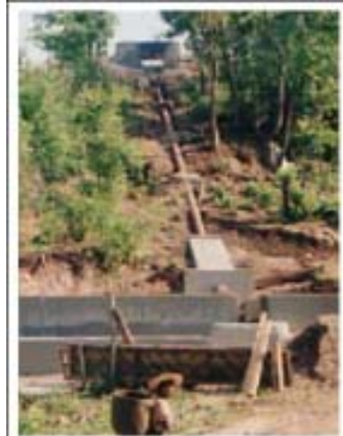
Anchor Block of Penstock
