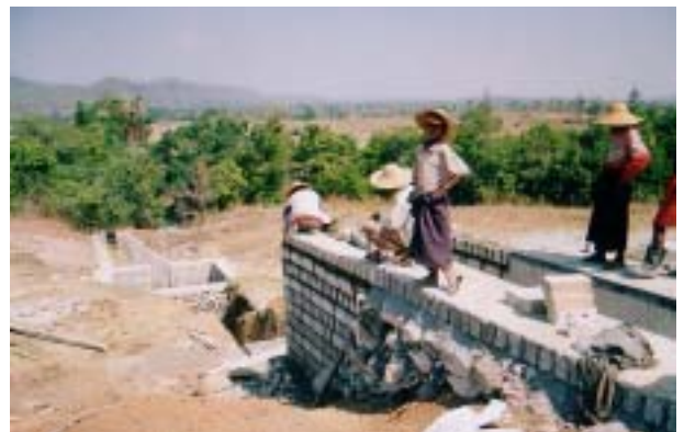
A sample of step spillway attached to the pond left.
