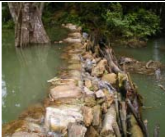
Sample of weir by sandbags
