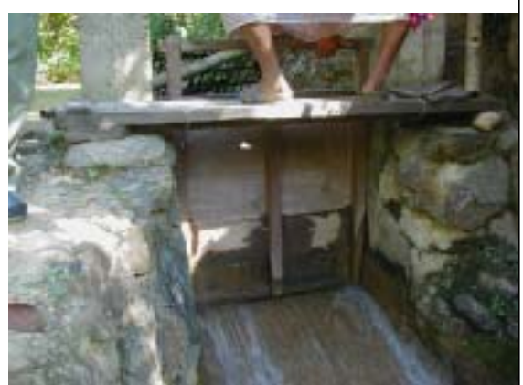
Wooden Hand-pull Gate Just start opening. The wooden gate well functions. Tha Le Oo.
