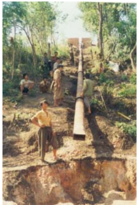
Construction on Self-Help: Waterways - Penstock (Pressure Pipe)
