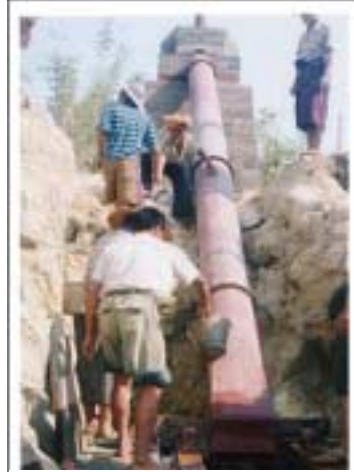
Penstock under Installation, Naung Bo
