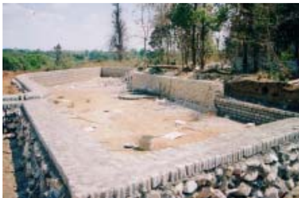
Stone masonry pond for villagers' amenity. It also functions as a head tank.
