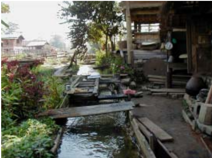
Village channel for Pico hydro
