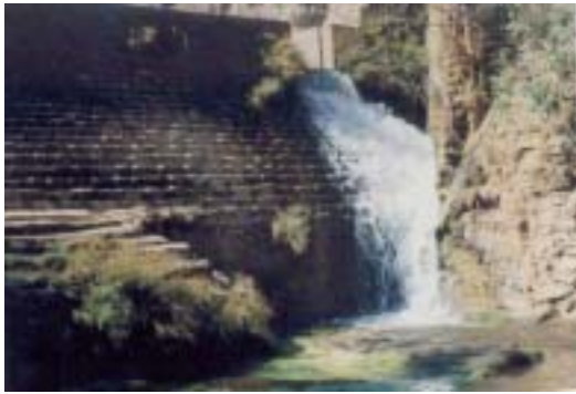
Sample of using existing structure Existing stone weir is used as intake.
