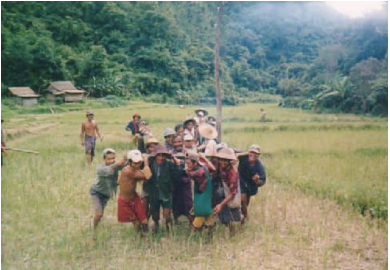
Construction on Self-Help: Transmission Lines
