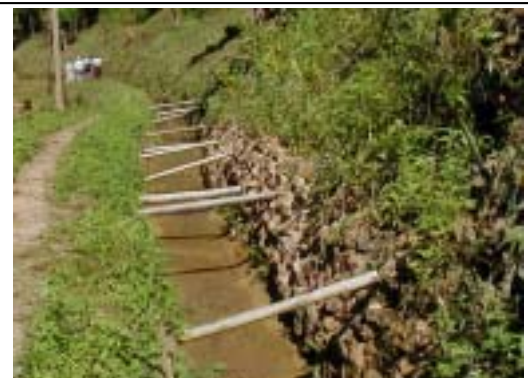
Power Canal under Construction, Tha Le Oo
